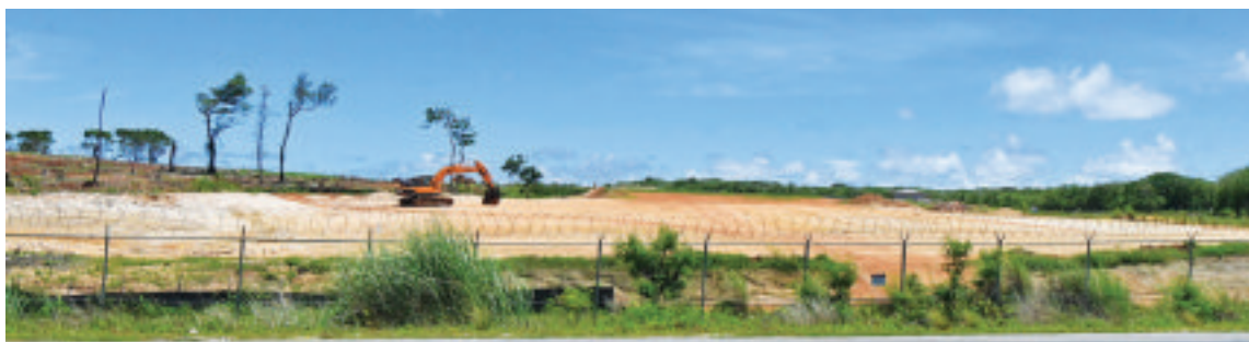
SITE WORK: Work continues to pave way for facilities within Marine Corps Camp Blaz which will host nearly 5,000 Marines who will be relocated from Okinawa. This was seen along Route 3 in Dededo on Sunday. David Castro/The Guam Daily Post
